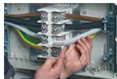
Conductor ends need to be rubbed with an acid and alkali free grease and immediately connected
