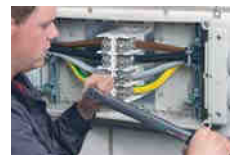
The terminals need to be tightened with the appropriate torque
