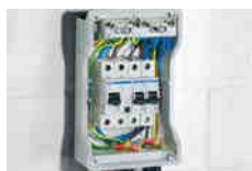
British Standard installation with earthed armored cables
