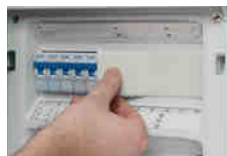
Blanking strips for unused DIN rail openings
