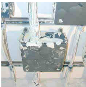
Junction box with connected cables after testing.
