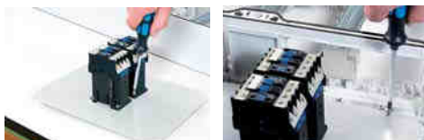
Device installation on mounting plates
